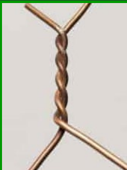
Correctly twisted wires should be even and look something like this.
